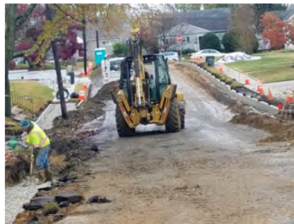
During repairs, construction crews seen working on new french drains.
